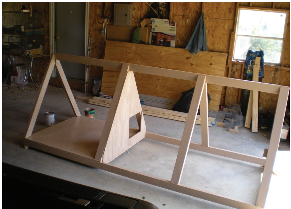
Figure 4. The ark frame before the wire and siding are added
