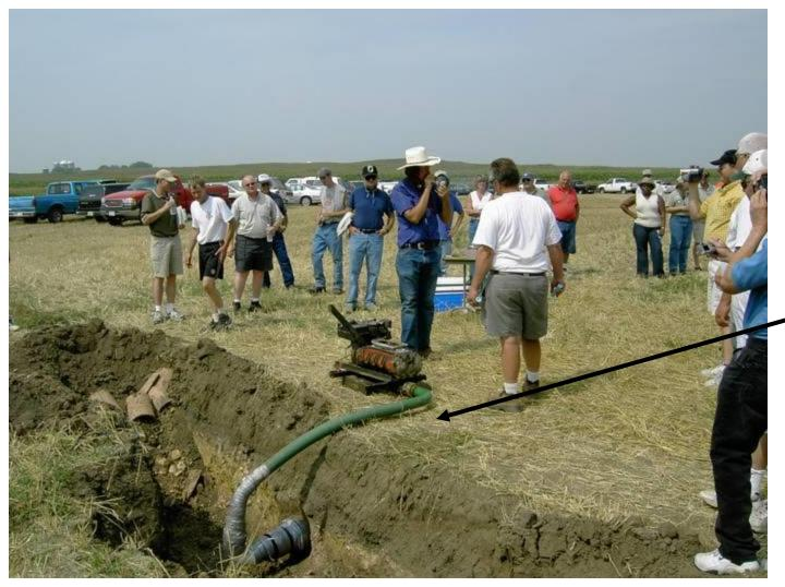
Smoke blower attached to tile line, immediately up from surface water outlet.
