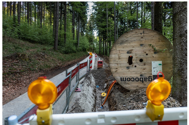
Broadband fiber installation
